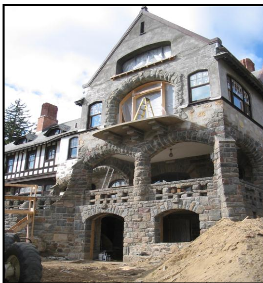
Photo 1 Second story addition (courtesy of OSHA)
