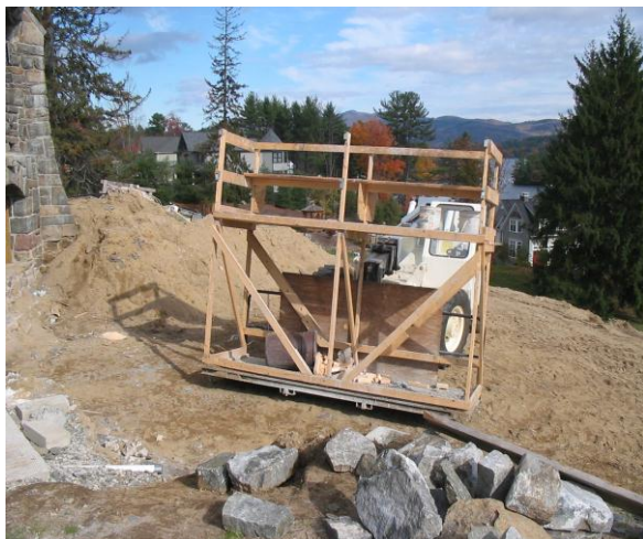
Photo 4 Two-tier Platform (courtesy of OSHA)
